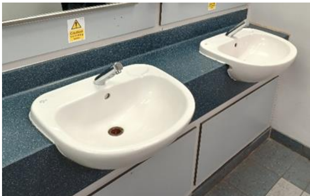
Sensor taps installed.
